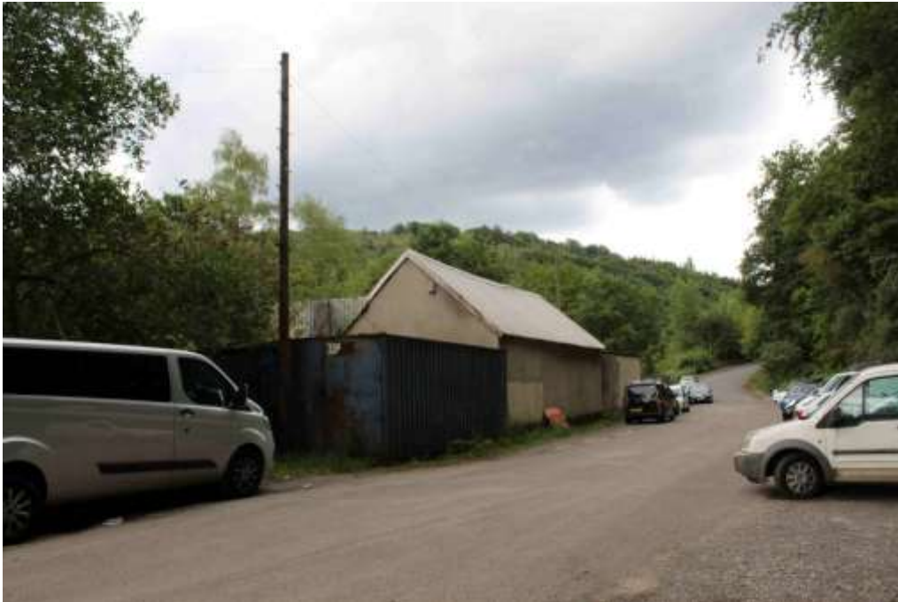
Plate 5. Listed Building: Former Navigation Colliery Group. View south-east towards the Site, from driveway.
