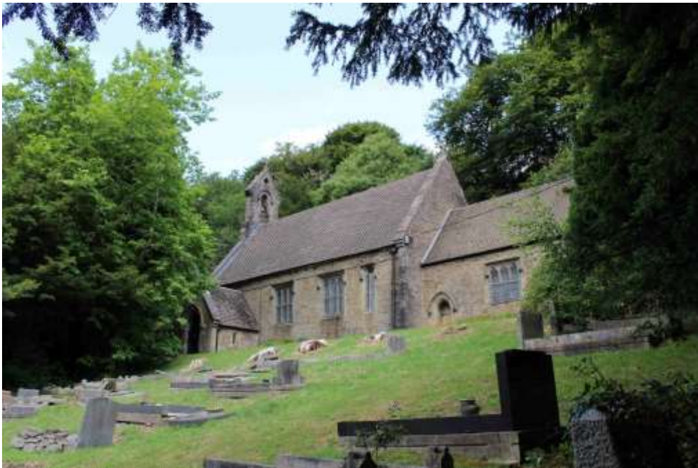
Plate 9. Listed Building: Welsh Presbyterian Church (Cadw 20995). View north-west
