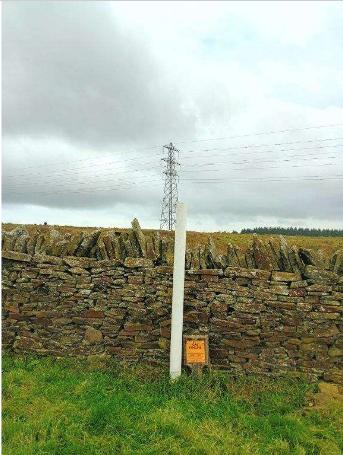
Plate 3: Gas pipeline marker post
