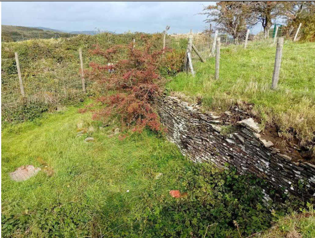
Plate 30: Field boundary between site and opencast operational site has masonry retaining wall ~1m (322810 , 196520) extent of wall not clear as area not accessible.
